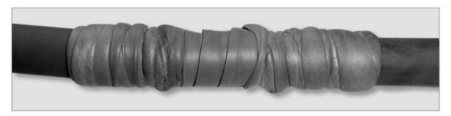
11. Use a glass sleeving, or something similar, to wrap tightly over the 2900 R tape to squeeze it right into the crimp link and into gap between the crimp link and the end of the insulation on the cable. After the 2900 R has been squeezed tight carefully unwind and remove the glass sleeving, then smooth out the surface of the 2900 R tape with your hand.
