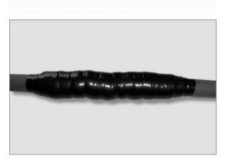
15. If you are joining single core to single core cables with staggered joints use a cold shrink over each individual joint.
