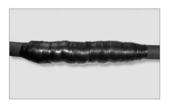
14. Lay 3 layers of Super 33+ electrical tape over the 130C tape with a half lap. Try to tape in an even and uniform manner to ensure a smooth and uniform shape, and that each layer is wrapped in the opposite direction.
