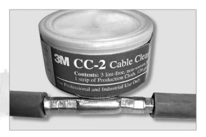
10. Lay 2 layers of 2900 R Sealing Collar Tape over the Crimp Joint and about 5mm over the ends of the cable with a half lap. Please ensure that each layer of tape is wound on in the opposite direction, i.e. if the first layer is wound left to right, the next layer should be wound right to left.
