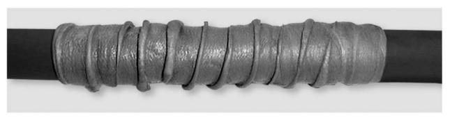
12. Lay 2 layers of Vinyl Mastic tape over the top of the 2900 R tape with a half lap as tightly as possible. Ensure each layer of tape exceeds the previous layer in length, and that each layer is wrapped in the opposite direction.
